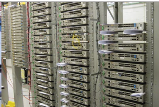
(Center) Switches for the VZW project are programmed in the lab before being deployed (Right) Splicing fiber
