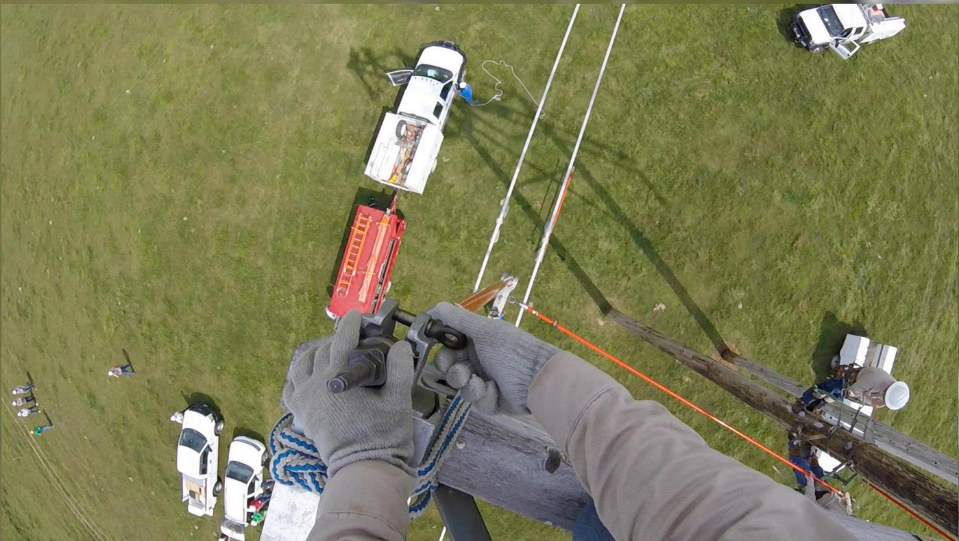
A view from the "hard hat cam" of Journeyman Lineman Ryan Huff as the Marshfield Line Crew performs a hot-stick procedure to change out a damaged insulator on a 345 kV line.
