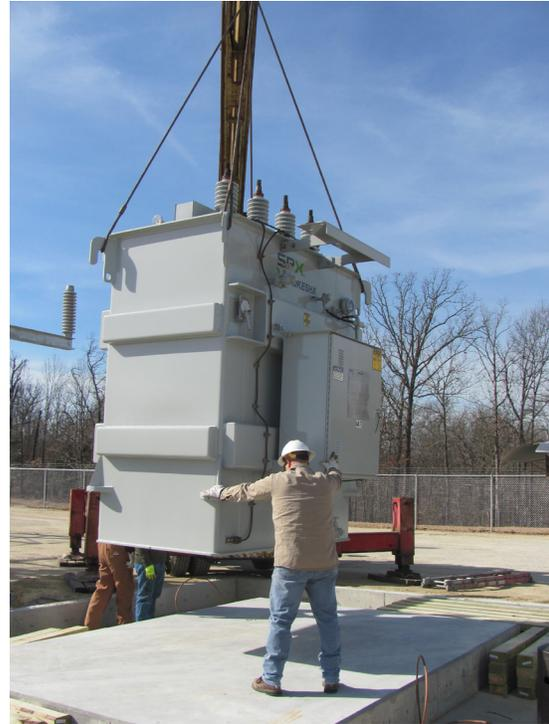
Substation Mechanic Craig Massey helps guide the 10 mVA transformer at Marshfield #5 substation onto its final destination.
