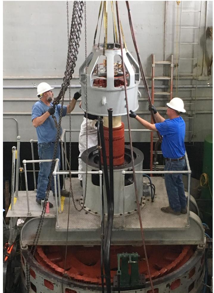
Substation Foreman Richard Newell and Substation Mechanic Chris Miller lower the rebuilt exciter onto the generator shaft of unit #2 at Tunnel Dam Hydro Generating facility.
